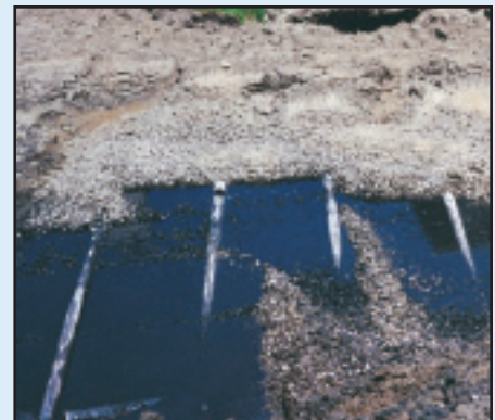
A failed system exposed.
