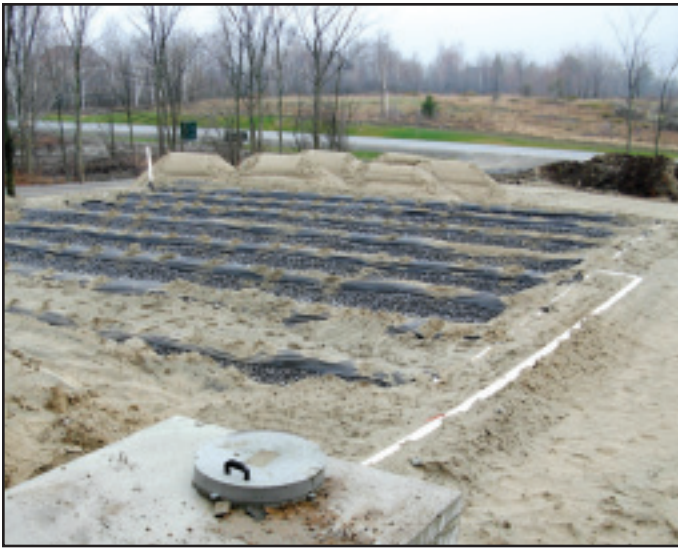
Leaching bed with perforated PVC drain pipes.
